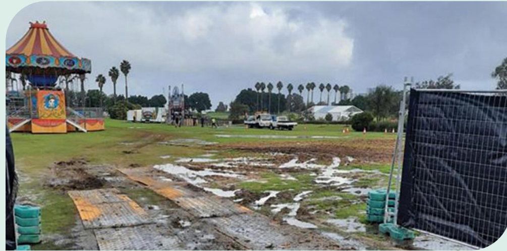
Earthworks and raising of South 9 site
